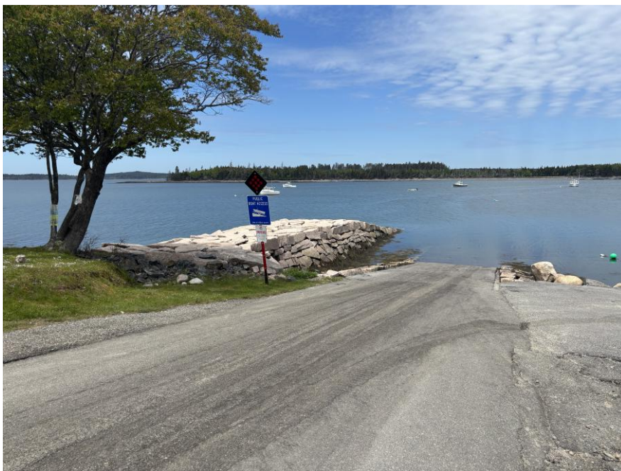
5 Pond Cove municipal boat ramp
